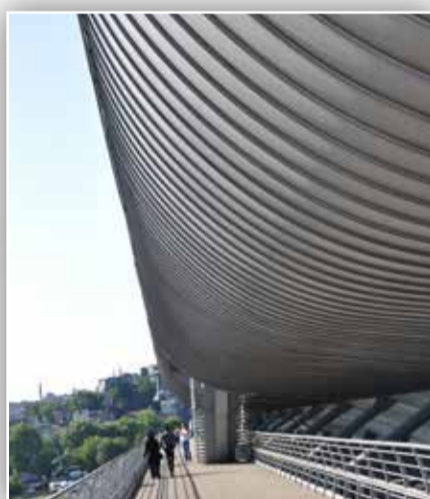
Location: Turkey Material: NedZink NOVA Architect: Hakan Kiran Architect Metal worker: Teknosel - Istanbul
