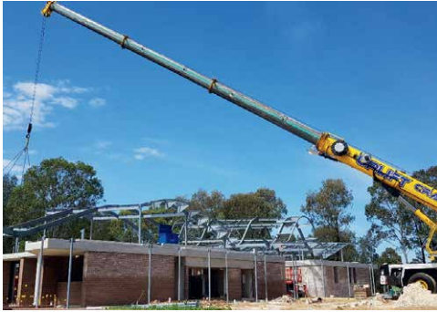
ABOVE: A construction scene at the centre, where the exposed skeleton of the roof shows the complexity in the design. CHS, RHS, SHS and EA in various widths were used to construct the shape, with no two pieces the same. (Image supplied by A Class Engineering.)
