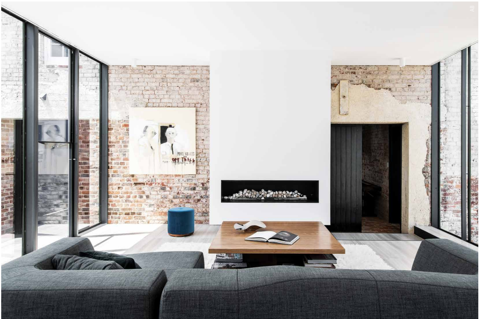
ABOVE: Inside the main living area in the new addition, spaces are kept open with custom fabricated slender steel mullions elegantly supporting the lightweight roof structure without the need for intrusive internal structural columns. BELOW: The rear wing of the existing Georgian building and its two symmetrical Georgian brick outbuildings have been connected and consolidated by a new lightweight glazed link custom framed with mullions fabricated from RHS.
