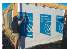
Fix securely to the frame with fasteners or tape.
