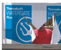
On arrival of doors and windows, cut Watergate at each opening on a 45° angle away from each corner. Pull the Watergate flaps inside and fasten to the inside of frame.
