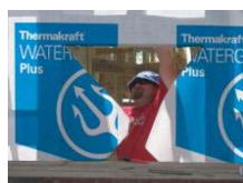
On arrival of doors and windows, cut Watergate at each opening on a 45° angle away from each corner. Pull the Watergate flaps inside and fasten to the inside of frame.
